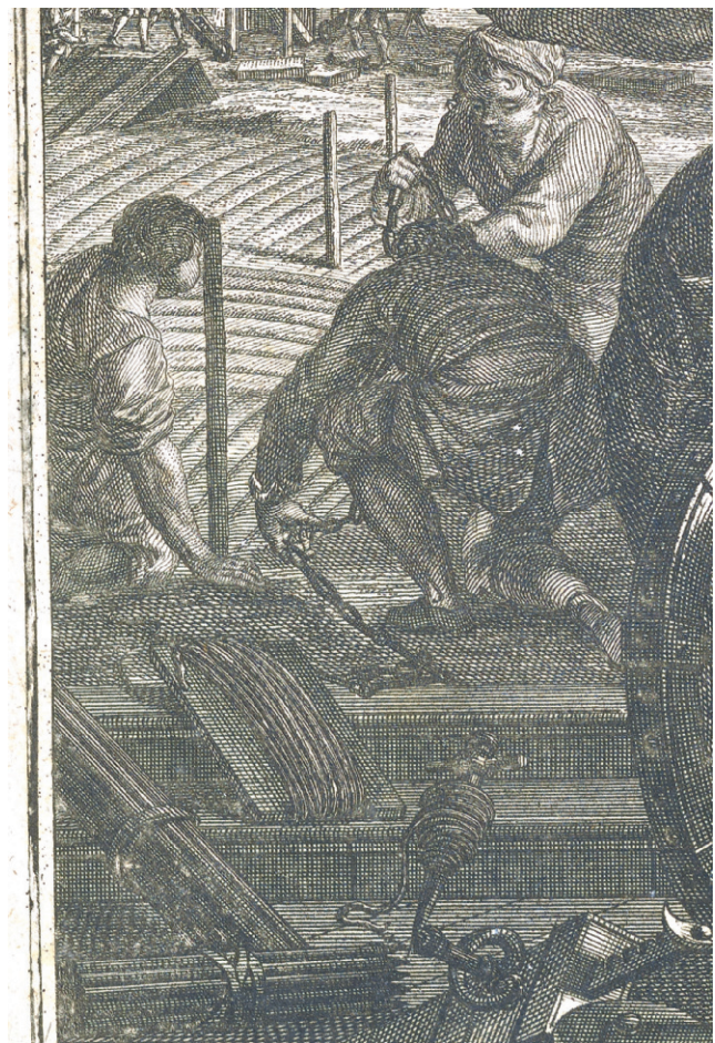
FIG. 414. SURVEYORS MEASURING A FIELD WITH A CHAIN. From Tobias Mayer, Mathematische Atlas, in welchem auf 60 Tabellen alle Theile der Mathematik vorgestellt (Augsburg: Johann Andreas Pfeffel, [1745]), frontispiece. In this detail note the use of stakes (also known as arrows or pickets) set up in a straight line to guide the chain. Image courtesy of the Osher Map Library and Smith Center for Cartographic Education at the University of Southern Maine, Portland (OS-1745-5).
