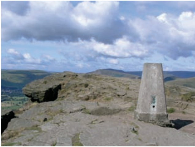
FIG. 773. ORDNANCE SURVEY TRIANGULATION PILLAR, WIN HILL TRIG POINT. Image courtesy of David Cotton, Cambourne.
