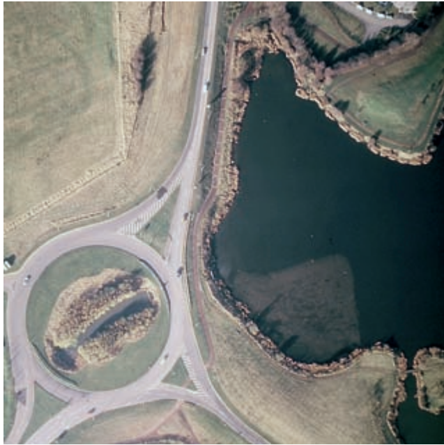
FIG. 688. COLOR AIR PHOTO OF A BALANCING LAKE NEAR MOUNT FARM LAKE IN MILTON KEYNES (U.K.), 26 NOVEMBER 1980. The balancing lake, which is used to control water levels in a river during periods of high rainfall, is important for environmental assessment and mapping. Copyright reserved Cambridge University Collection of Aerial Photography.
