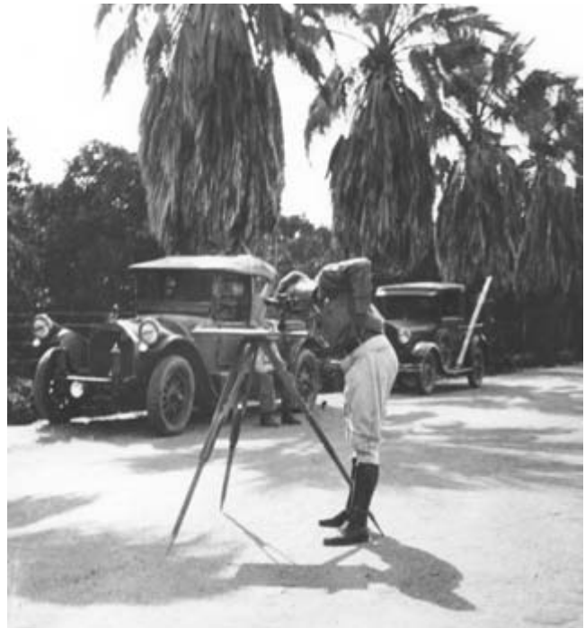
FIG. 988. SURVEYING WITH PLANE TABLE AND ALIDADE. USGS topographer George Stanley Druhot in Fullerton, California, 1932. In the second car behind Druhot, a stadia rod is visible.
